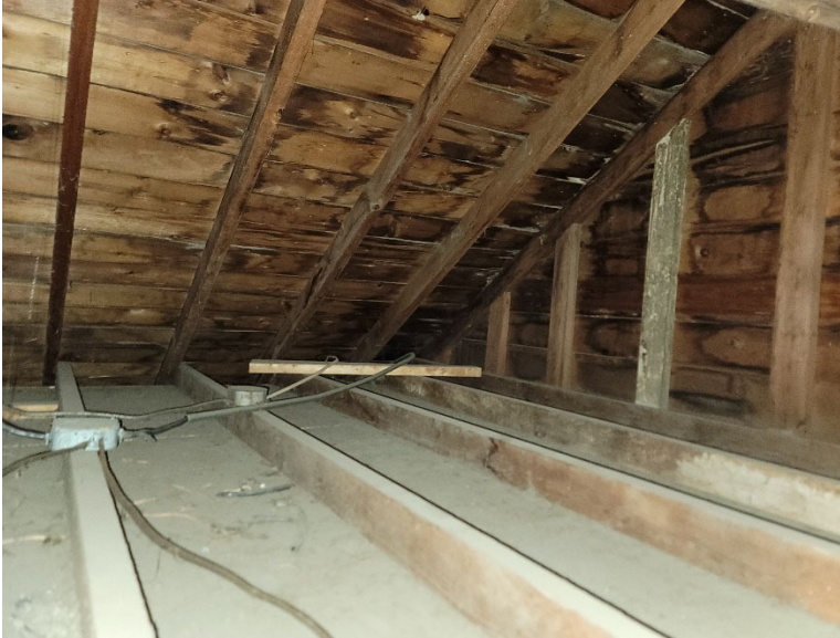
Figure 7 Area above rear portion of building
