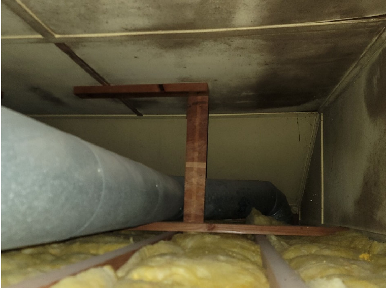
Figure 9 Original panel ceiling on roof joists
