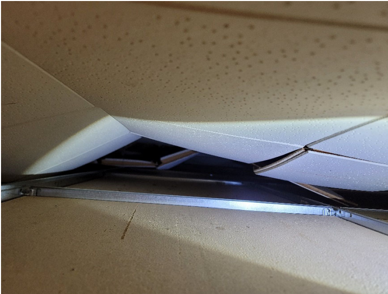
Figure 8 Area above Community Room ceiling
