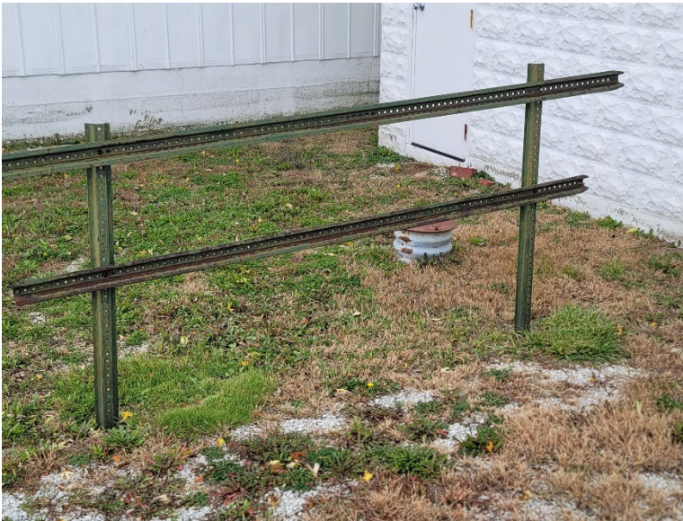
Figure 6 Septic tank cover
